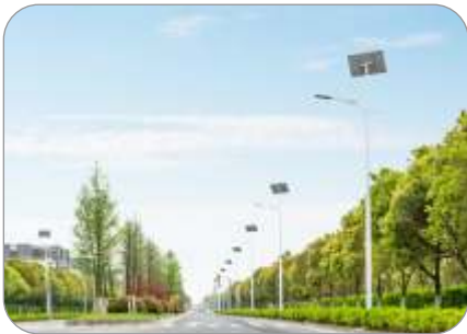
SOLAR POWERED STREET LIGHTS
